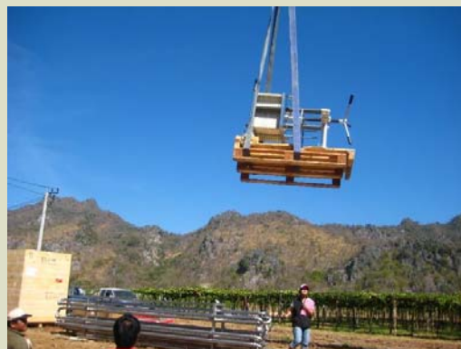
Lifting in a new filter, vineyard in the background
