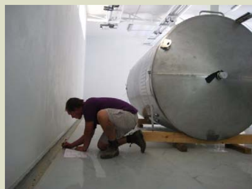
Tim Bartsch marking out the tank's position
